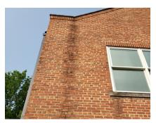
age. No signs of structural distress were observed. There were a few areas where mortar had begun to chip/crack and a few window heads where lintels could be observed. Recommend engaging a contractor experienced with treatment of historical buildings to perform a cleaning of the overall building exterior followed by tuckpointing or repointing, as appropriate. As part of this work, it will be important the contractor utilize materials and techniques
