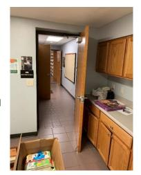
Generally speaking, all doors in use by the public must have 1'-0" of clearance beside the door on the push side and 1'-6" on the pull side with less than an 8-inch recess in the wall. Some doors are significantly recessed in the wall and will require modifications to meet the required clearances.
