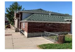
The main building has a sloped asphalt shingle roof in a hip configuration. The former car port and park shelter roofs are also asphalt shingles in him configurations that tie into the library building. The shingles and roof intersections appear to be in good condition and there was no visible evidence of deterioration.
